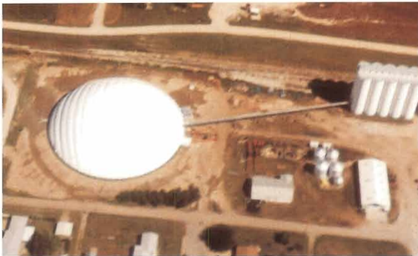
Farmers Co-Op Elevator Dighton, Kansas 252' Diameter x 63' High Clear Span
