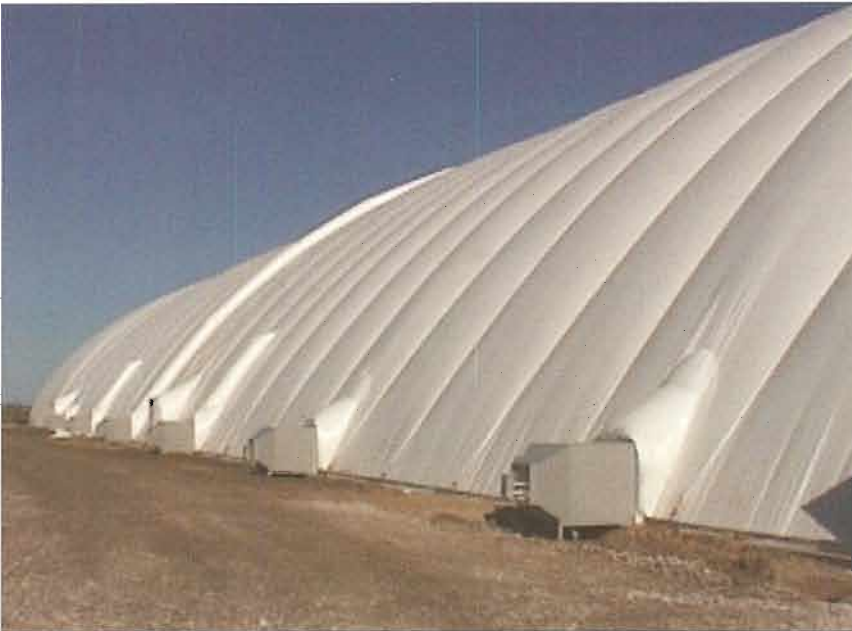
Featuring a bank of six Air Filter Vents down the side of the structure to improve the air quality inside the dome
