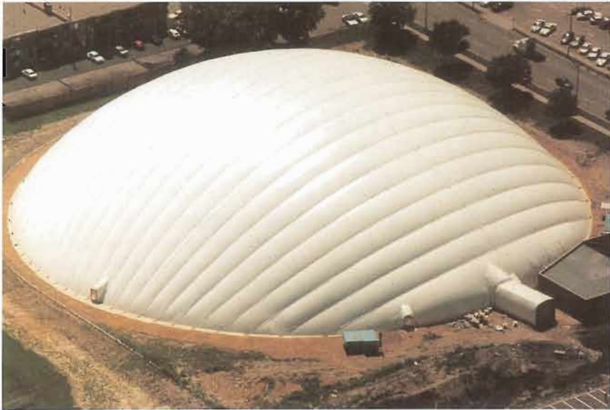
RICE & ARLINGTON SPORTS DOME 360' Diameter x 90' H Round Structure St. Paul, MN
