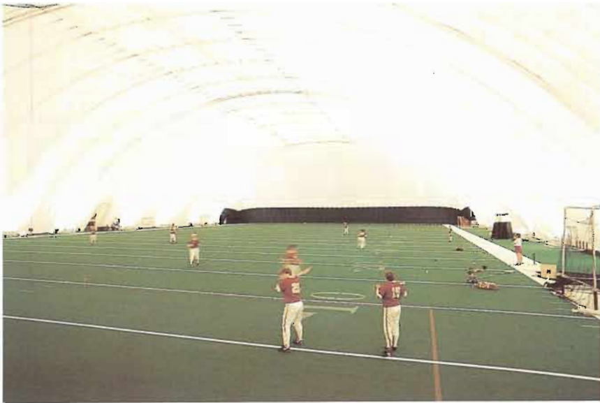
Interior is illuminated by protected floor mounted metal halide lights, providing indirect lighting to the playing area.
