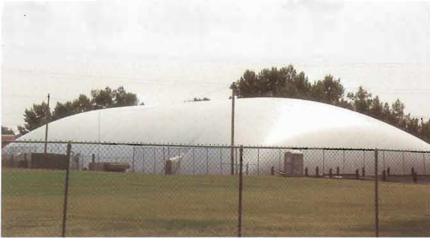
Rico Tennis Academy 4 Court tennis – membrane replacement Calgary, Alberta
